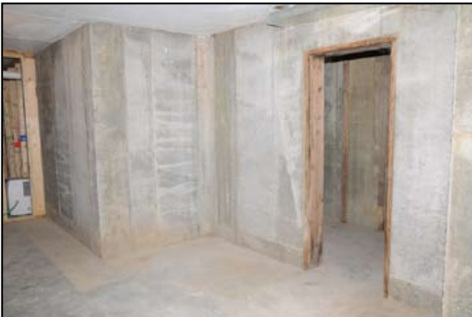
View Of Basement Looking Toward Storm Shelter
